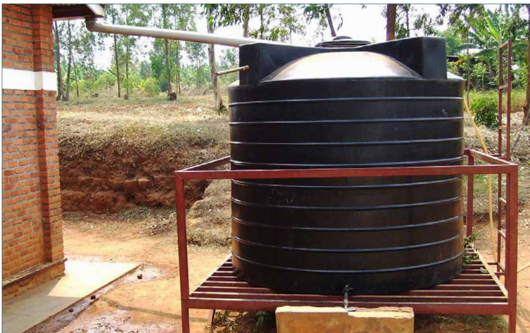
Rebates are available on tanks like these that can store rainwater for use during drier months.
